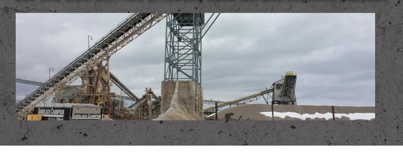
Scope: This project involved temporary steel shoring, demolition of existing steel structures, new steel erection, grounding of base plates, and concrete saw cutting. Gundlach Champion provided all labor, materials, and equipment required for the modifications.
