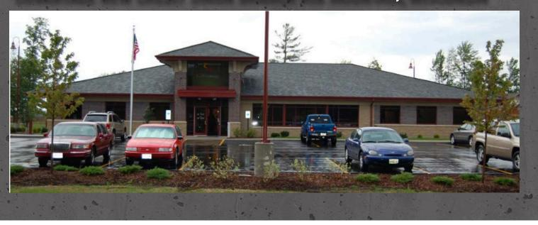
**Scope:** The project consists of a 7000 sf, slab on grade, wood frame / brick veneer structure. The roof is wood truss with asphalt shingles and skylight. Interior is metal studs and drywall with carpet / ceramic tile flooring, acoustical ceilings, paint & vinyl wall covering, plastic laminate casework and standard plumbing, HVAC and electrical packages. Exterior concrete curbs & walks, landscaping and asphalt paving are also included.
