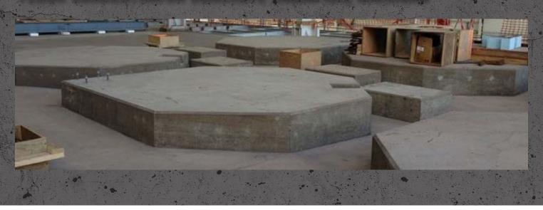
**Scope:** This project consisted all excavation and backfill along with forming and placing 6,000 cyds of concrete foundations for process equipment, an elevated electrical room, transformers and switch gear, 40,000 sq. ft. of slab-on-grade, miscellaneous handrails, anchor bolt setting.
