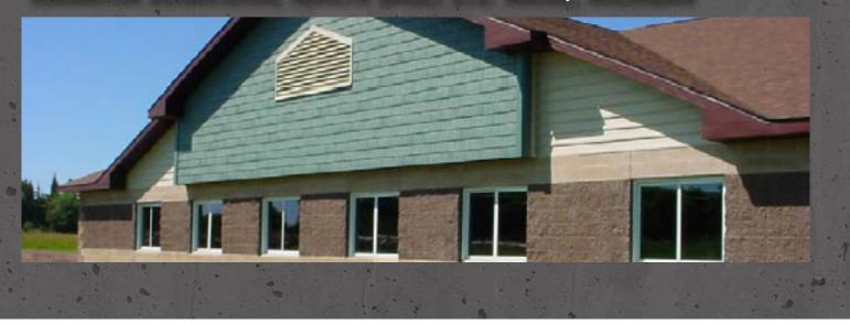
**Scope:** Negotiated with GMP, self-performed concrete, masonry, structural steel and carpentry. This 24,000 square foot new office and clinic consists of a wood frame with split face masonry exterior. The clinic houses approximately sixty suites, several conference rooms, and a kitchenette and break room, along with clinic areas. In addition to the building, construction also included a lighted parking lot. The project was completed on time and under budget.
