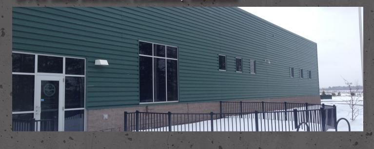
**Scope:** Gundlach Champion was the General Contractor on this new 11,000 sqft combination masonry / structural steel studs bearing structure. The facility includes a grain storage vessel, loading dock area, brew house, fermentation room, keg and bottle line, and tasting room. Flooring in the brewing area consists of quarry tile with integrated trench drains for ease of cleaning. This facility will distribute product across Michigan's Upper Peninsula and adjacent states.
