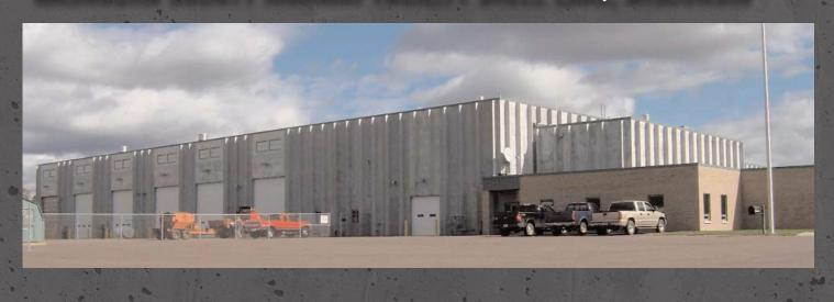
**Scope:** This Construction Management project is a new one story, 75,000 square foot highway facility which includes office areas and a conference room in addition to locker room facilities. The garage area includes storage for approximately 50 vehicles, wash bays, repair bays, parts storage area, a sign shop, overhead crane, vehicles lifts, and lube dispensing equipment.
