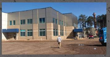
items from its wish list, they were able to work within their project constraints. Because the building was designed with precast concrete walls, GCI was able to expedite the production and installation of the panels to ensure the project stayed on schedule.
